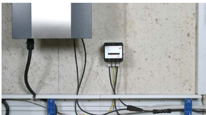
Prewired connecting cables for easily connecting the incoming string lines to DEHNCube and the inverter.
