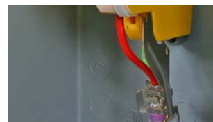
EMC spring terminal (accessory) for permanent low-impedance shield contact.
