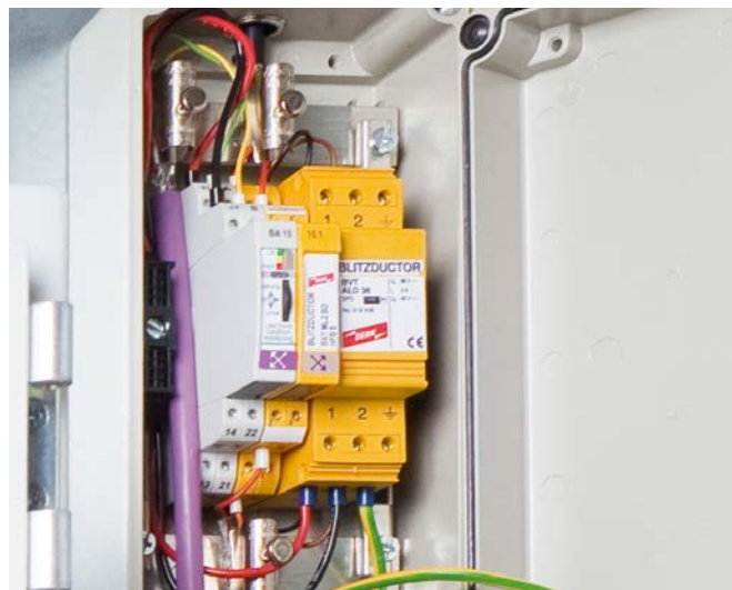
Compact DIN rail mounted surge protective device with screw terminals for stranded lines.
